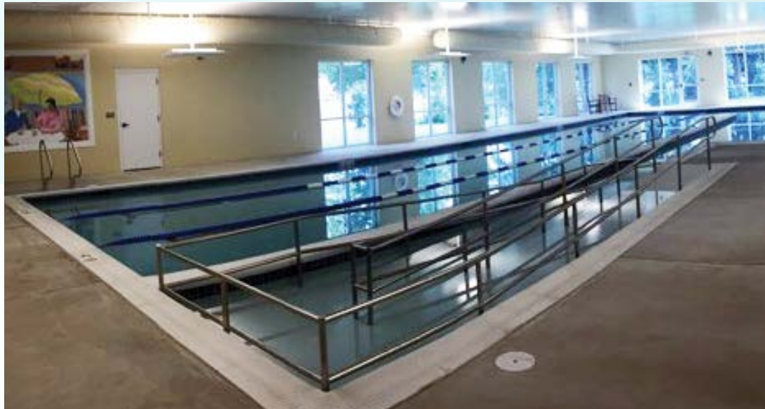
Indoor Heated Pool
